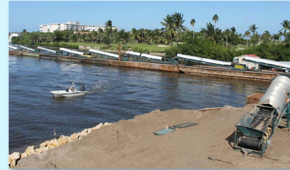
Figure 6: Conveyors transporting sand from island stockpile to sand shooter.
