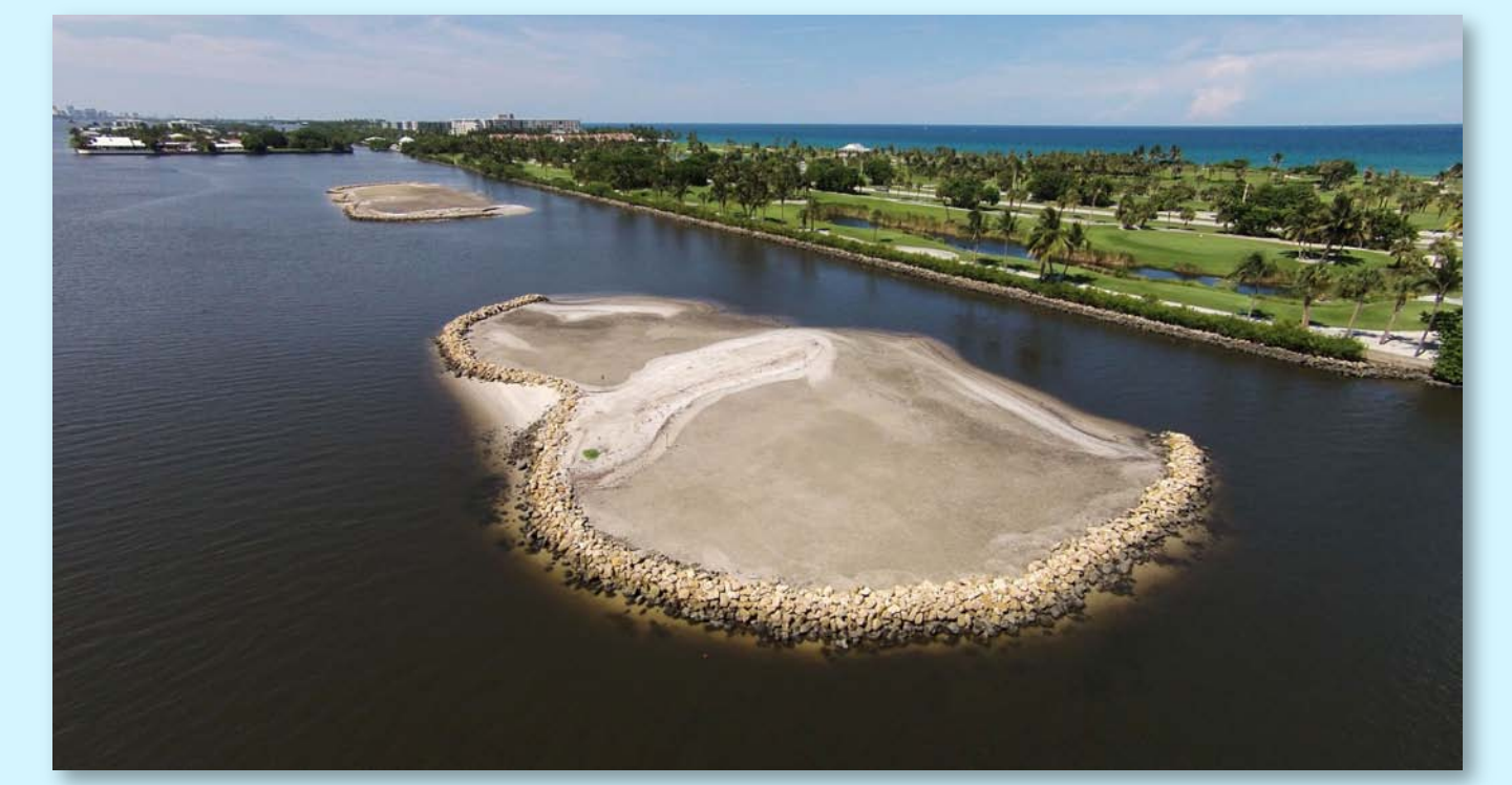
Figure 12: Grassy Flats post construction.
