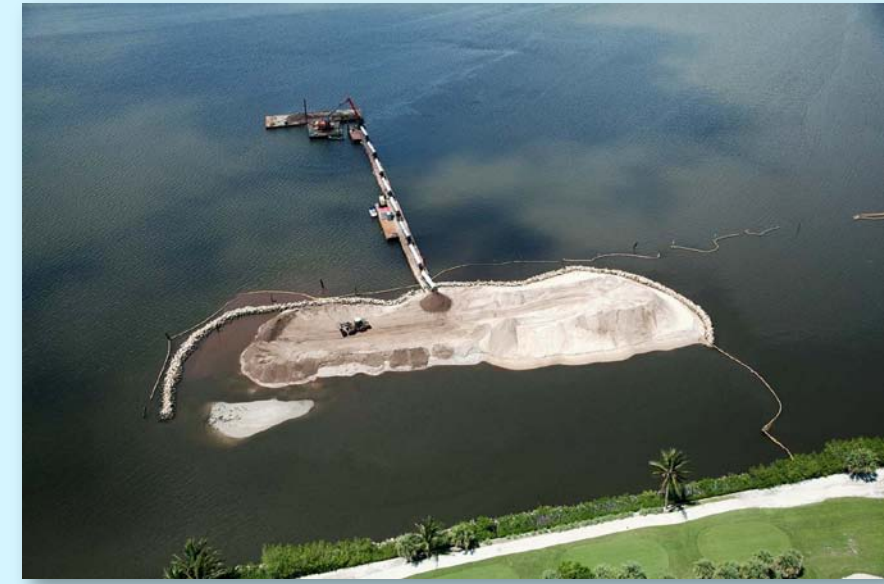
Figure 5: Unloading sand from barges using conveyor belts. Photo Credit: Eastman Aggregate Enterprises, LLC and Smith Aerial Photos.
